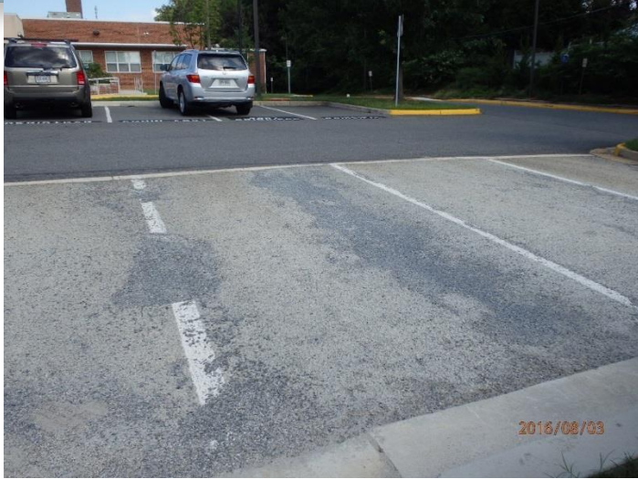
Deteriorated Porous Concrete Replaced with Porous Concrete Slabs
