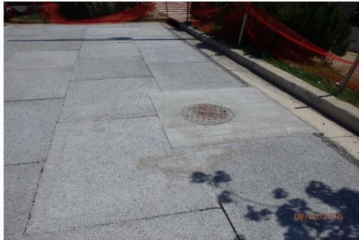
Deteriorated Porous Concrete Replaced with Porous Concrete Slabs
