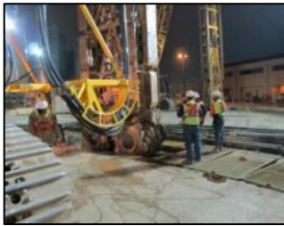
Slurry Wall Construction
